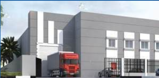
Project: G+M Warehouse & Office
