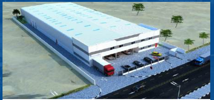
Project: G+M Warehouse & Office
