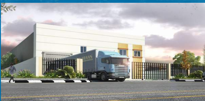
Project: G+M Warehouse & Office
