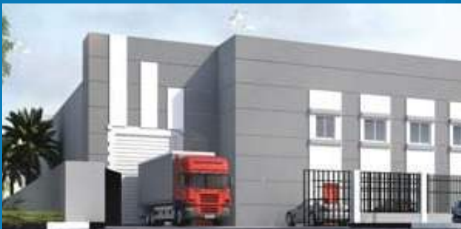
Project: G+M Warehouse & Office
