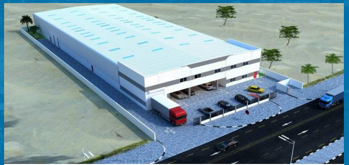
Project: G+M Warehouse & Office
