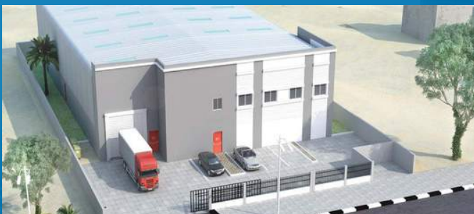
Project: G+M Warehouse & Office
